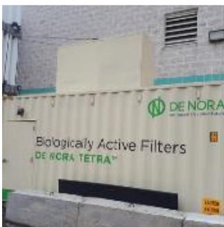
Combining ozone with a biologically active filter (BAF) in a drinking water plant is a cost-effective way of dealing with contemporary drinking water sources without using membranes or other technologies that produce difficult-to-dispose concentrate streams. Ozone mainly breaks down the large organic molecules in the source water and is then followed up with a biologically active filter to remove the remaining contaminants.
